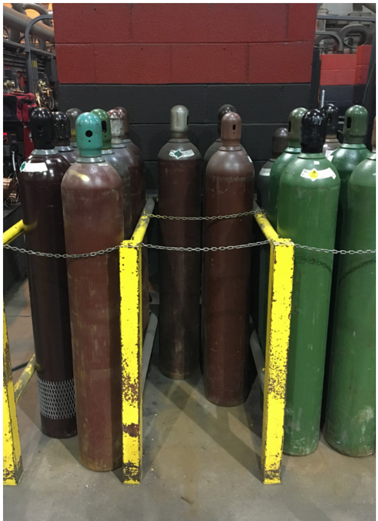
Figure 2-15: Inert Gas Cylinder Storage
