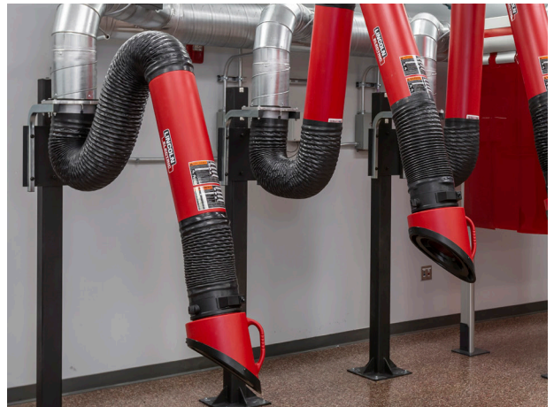
Figure 2-17: Centralized Fume Extraction Arms
