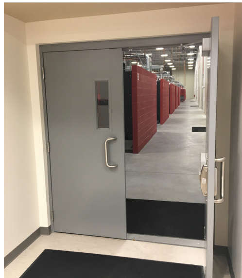
Figure 3-2: Large Double-Door Entryway
