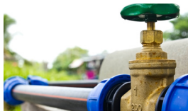
SOLDER WATER PIPES
