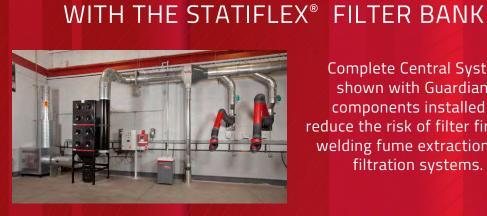
Complete Central System shown with Guardian™ components installed to reduce the risk of filter fires for welding fume extraction and filtration systems.
