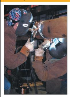
10 inch / 6 inch (254 mm / 152 mm) pipe in pipeline for the North Sea utilizing the STT process together with Outershield gas-shielded flux-cored wire. Tie-in welds on the Williams Devils Tower project and BP King West project in the Gulf of Mexico will also be using Outershield wire.
