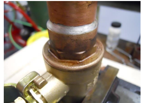
4 To ensure good penetration : (a) Watch for solder to melt when applied . It should flow into the joint . If it just lays on top the parts aren't at the correct temperature. (b) Direct flame to valve base to pull solder into the joint.
