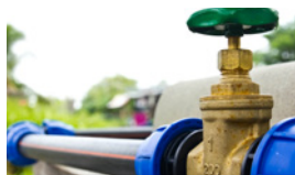
SOLDER WATER PIPES
