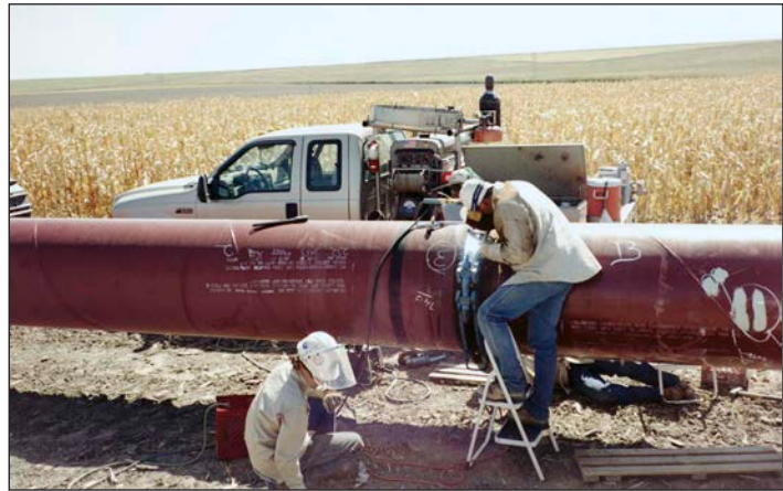
Cross-country pipe welding.
