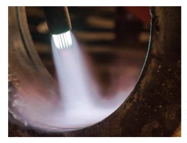
The easiest way to prevent underbead cracking is to slow the cooling rate by preheating.
