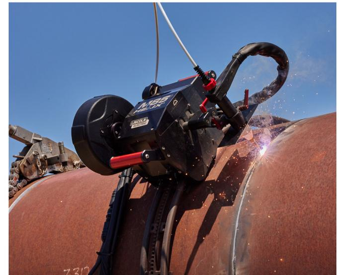
(1) Advanced process MIG modes (Pulse and STT Field) available with use of Activ8X Pipe Wire Feeder
