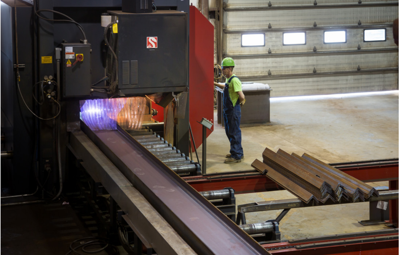
PythonX processing a structural steel beam
