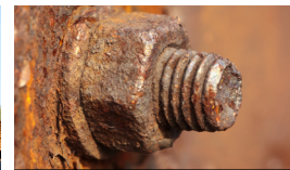
CUT OFF A RUSTED BOLT
