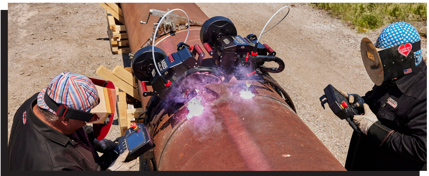
Two AutoShield set-ups welding in the field
