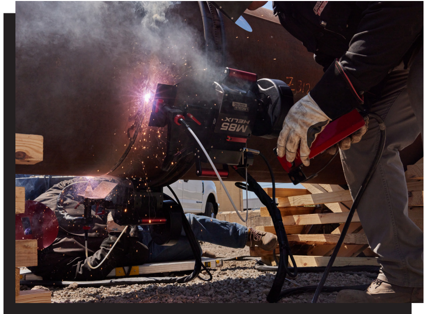
Two AutoShield set-ups welding in the field
