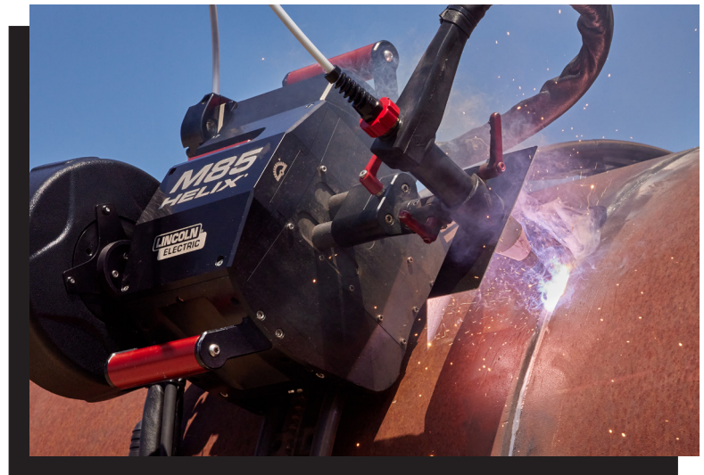
The AutoShield orbital welder in motion
