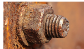
CUT OFF A RUSTED BOLT
