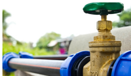
SOLDER WATER PIPES
