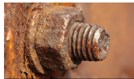
CUT OFF A RUSTED BOLT
