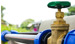
SOLDER WATER PIPES
