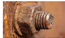
CUT OFF A RUSTED BOLT
