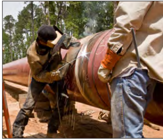
Cross-country pipe welding.
