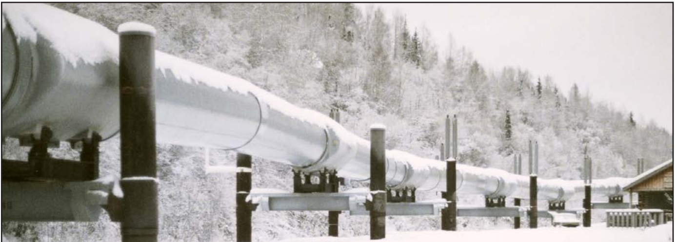
The 800 mile long 48 inch diameter Trans Alaska Pipeline System was constructed using Lincoln Electric Pipeliner® welders.
