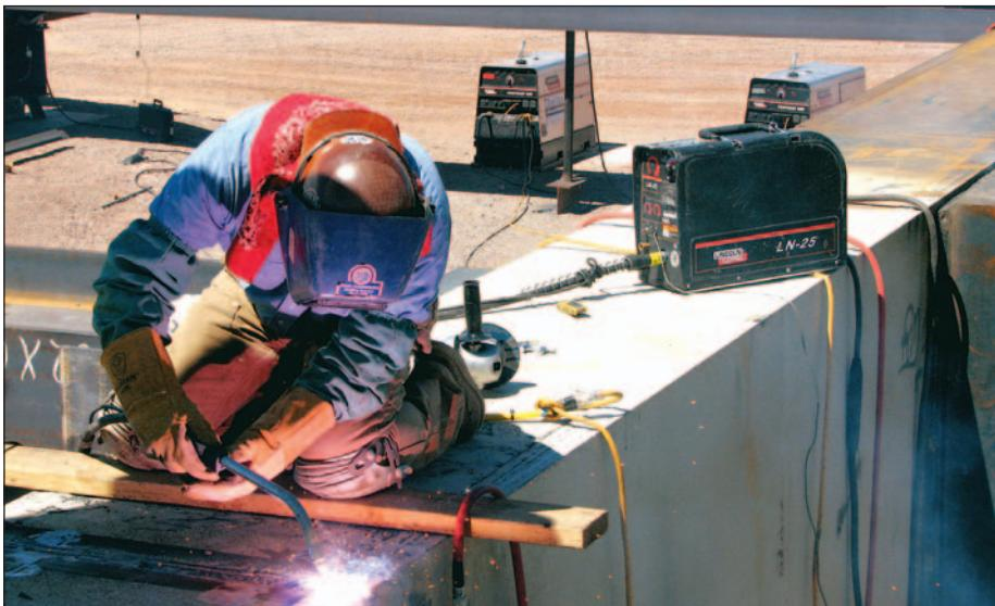
The shops fabricators had typically beveled material of this size 30 degrees on each edge to form a combined 60-degree bevel at the joint. Now with greater penetration abilities, the bevels have been reduced to 22.5 degrees at each edge to form a 45-degree total wedge.
