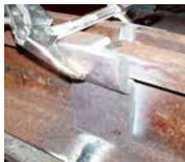
Rail web welding
