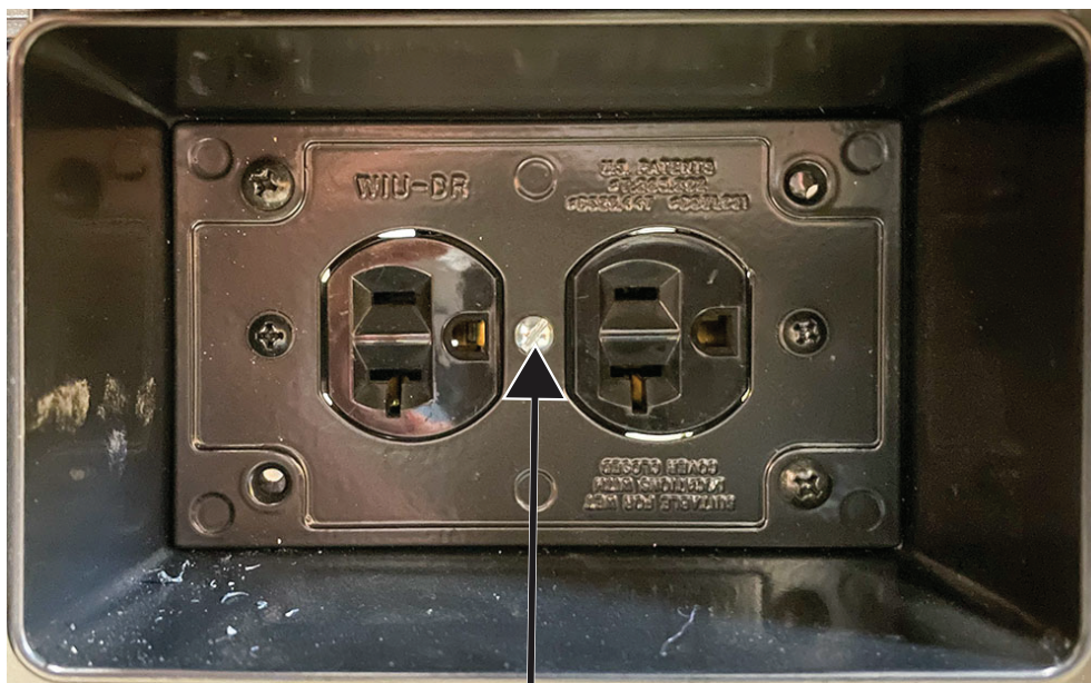
Figure F.4 – 120 VAC receptacle mounting screw location
