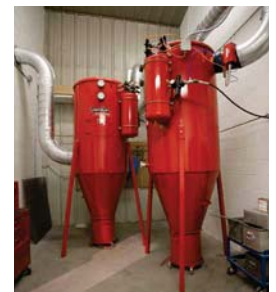
Eastern Wyoming College utilizes a high vacuum central system for fume extraction.
