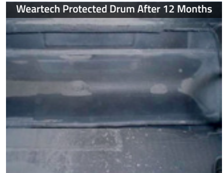
Vane pockets show minimal wear and no corrosion damage.
