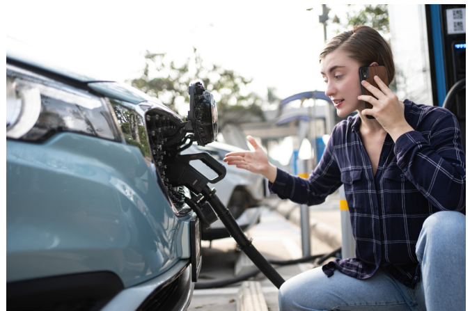
Broken electric vehicle charger leads to maintenance calls.
