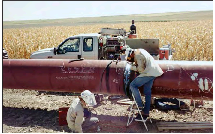
Cross-country pipe welding.
