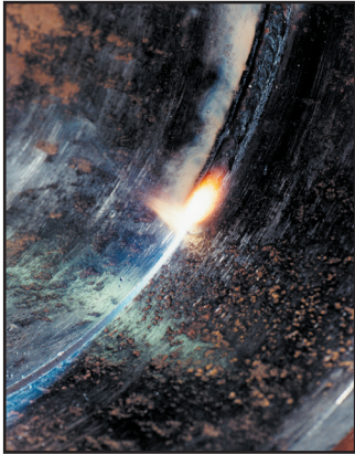
Inside of an 8 in. x 0.375 in. wall API 5L-X52 pipe, welded in 5G position.
