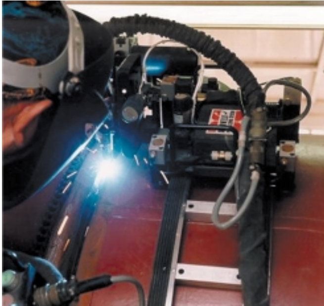
The STT in the Autoweld system.
