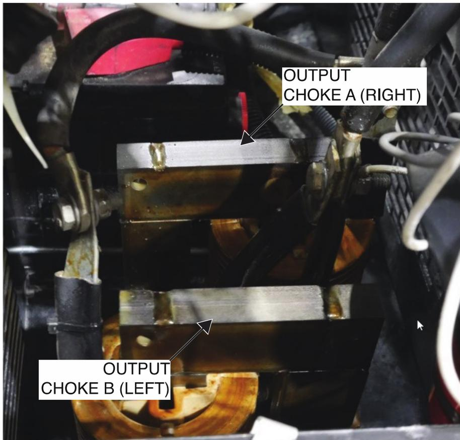
Figure F.2 – Output choke lead locations
