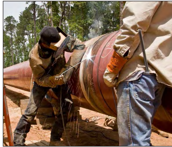
Cross-country pipe welding.
